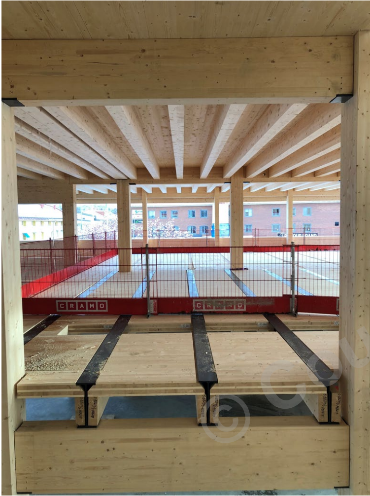
Hybrid steel timber floors
